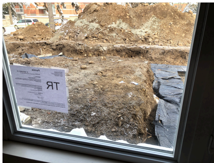
Construction at the shelter
