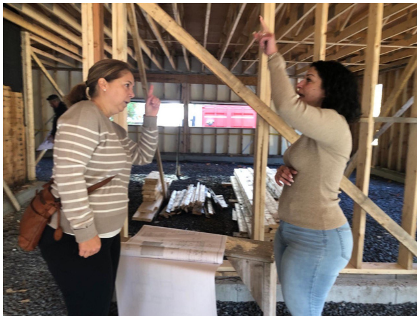
Construction at the shelter
