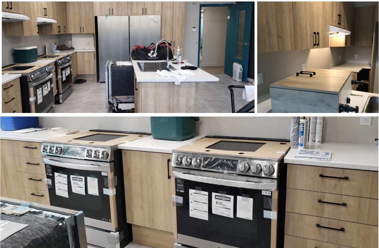
Construction at the Second Step Resource
